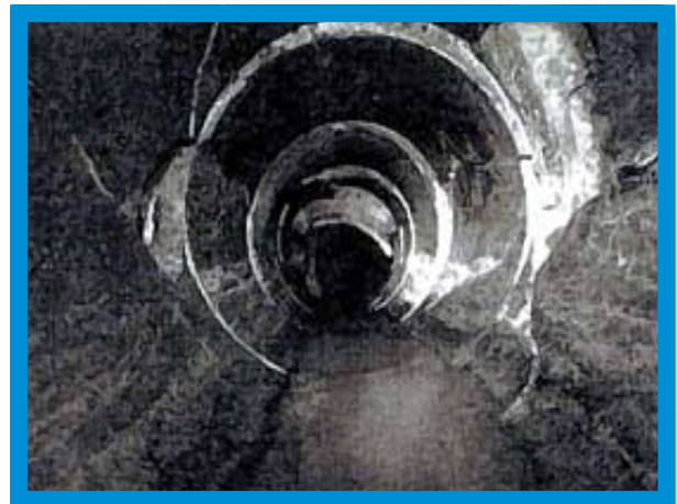
Cracked / Fractured Pipe
