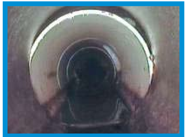
Cracked / Fractured Pipe
